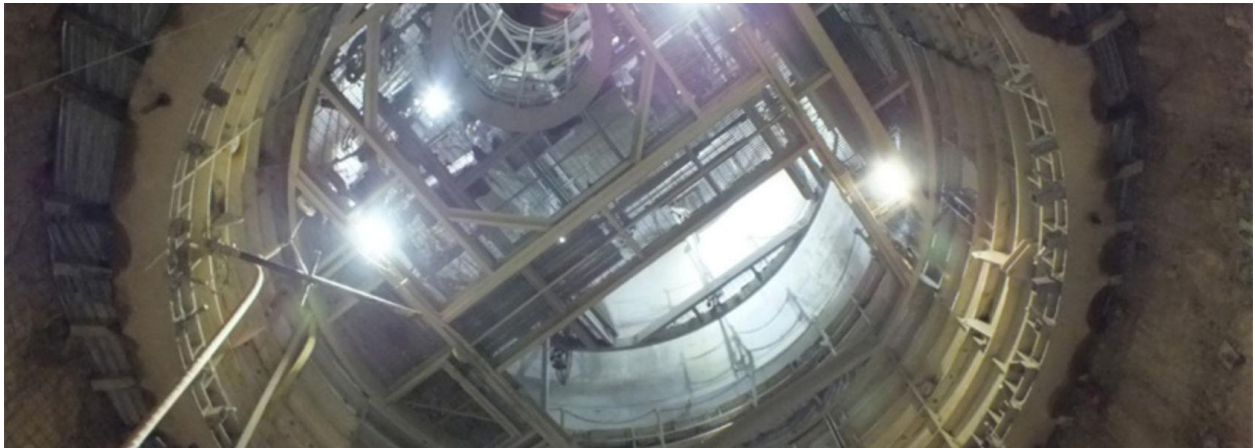
Looking up through the shaft at Nevada Copper's Pumpkin Hollow project
