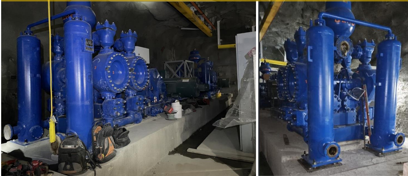
Geho Dewatering System – Mechanical Completion
