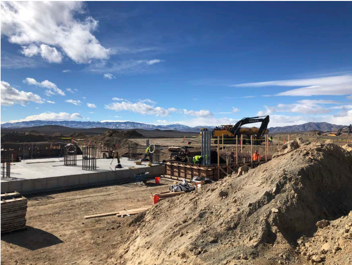
Sag/Ball/Verti Mills and Cyclone Foundations well Advanced
