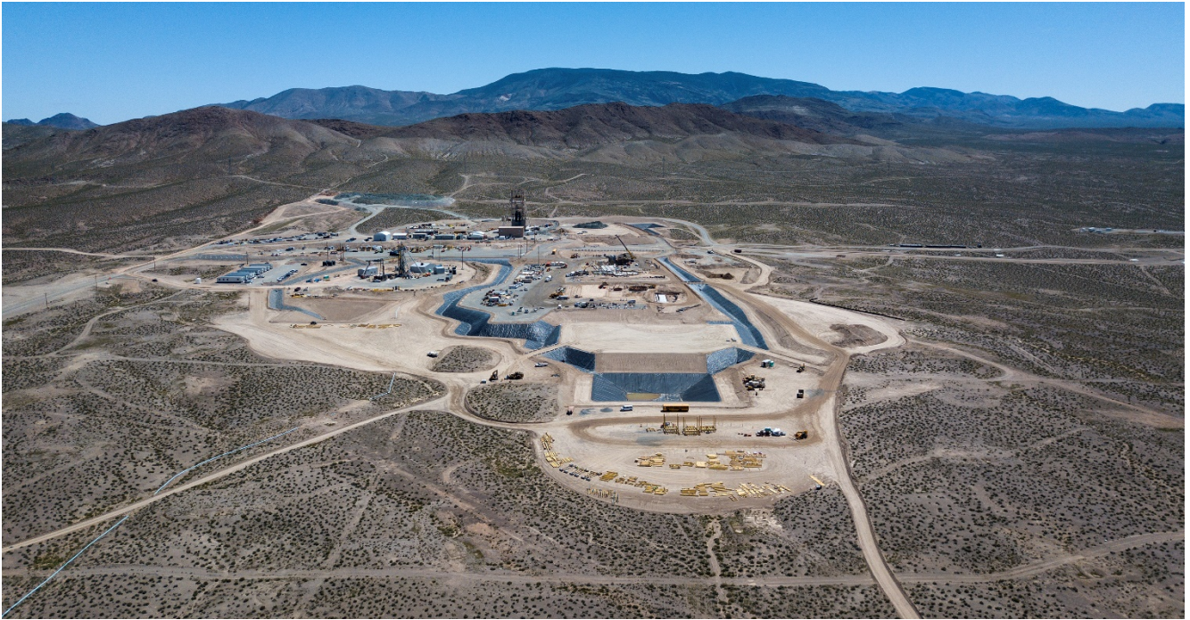
(Pumpkin Hollow Underground Project looking East)
