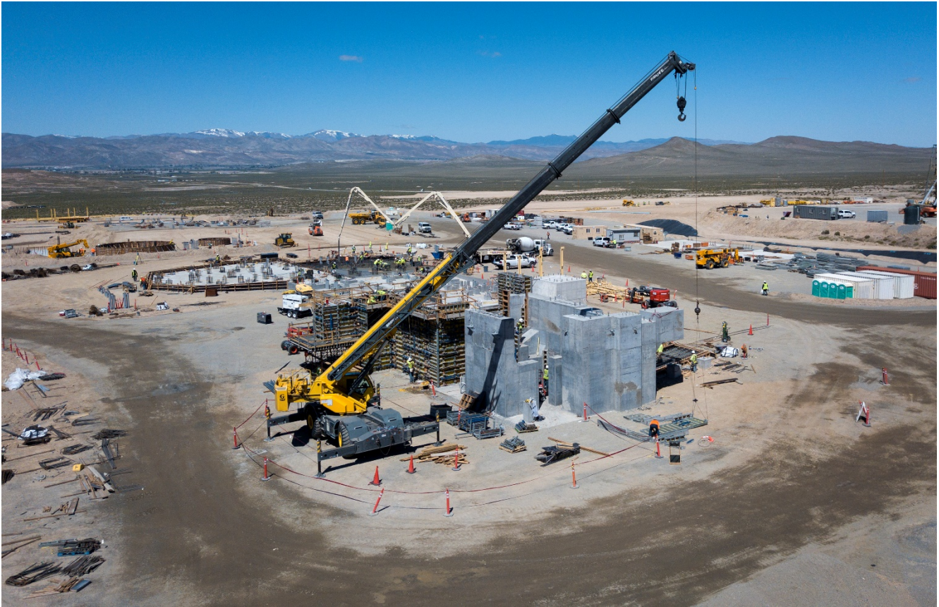
(Sag & Ball mill pedestals completed)
